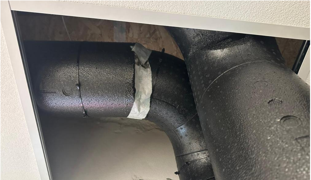
Figure 6 - Air leakage in EPP ducts
