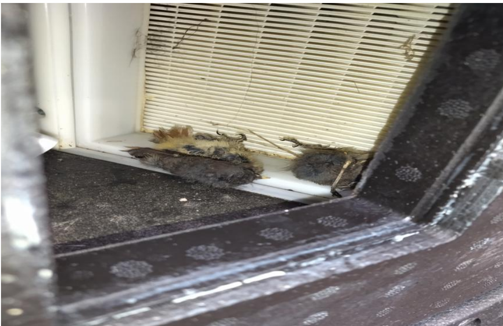
Figure 3 - Contamination of the heat exchanger space
